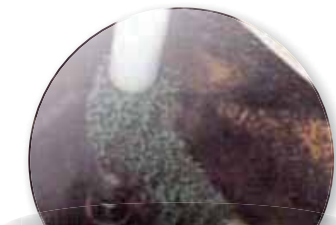
When light penetrates in the tank : Moss and microorganism grow.
